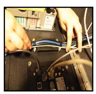
**10.**) Clean up the Loose harnessing and cords using the preexisting Clips and cable ties. Best practice to keep kiosk cabinet Clean.
