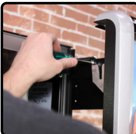
2.E) Pull out upper slide and mount to door. Install nuts loosely.
